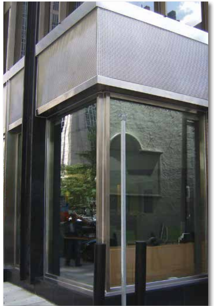
TD Bank Front – Boston, MA C 1008 Pyramid (Nickel) Elkus Manfredi Architects – Boston, MA
